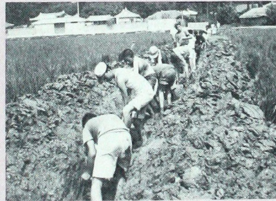
Students digging trench for irrigation pipe
