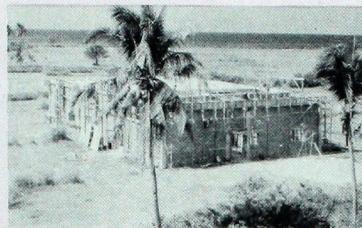
Station DWRP under construction
